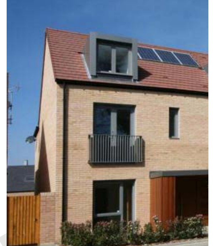
Simple Balcony on House overlooking a Green Space and Square Dormers
