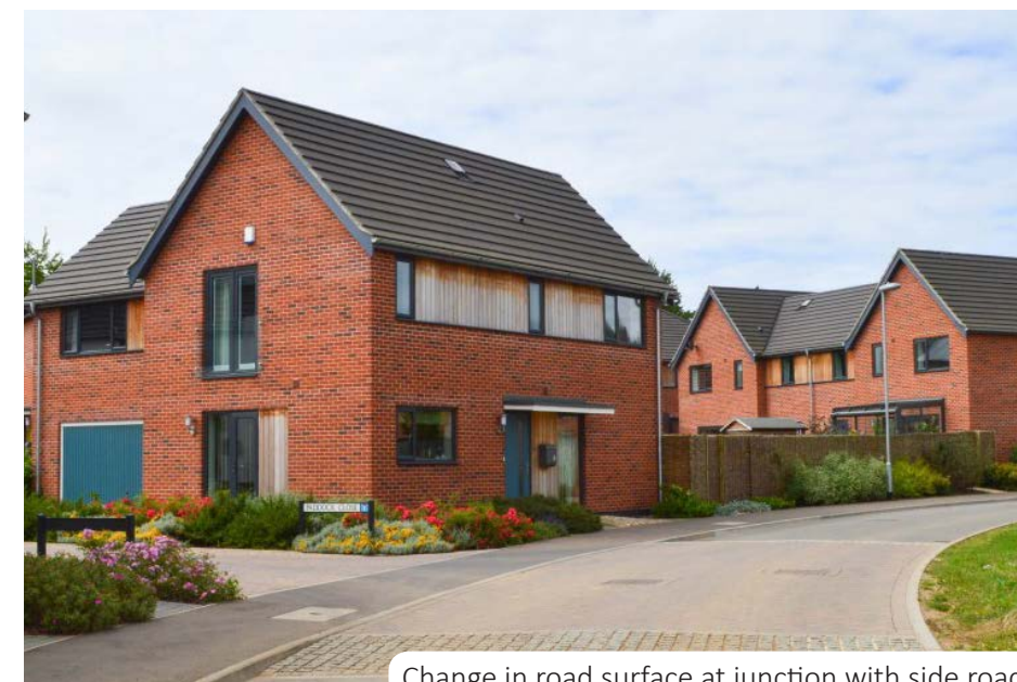
Change in road surface at junction with side roads
